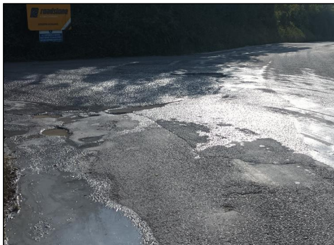
Photograph 11: View South of Potholes on East Edge of L1222 at Roadstone Joseph Hogans Quarry
