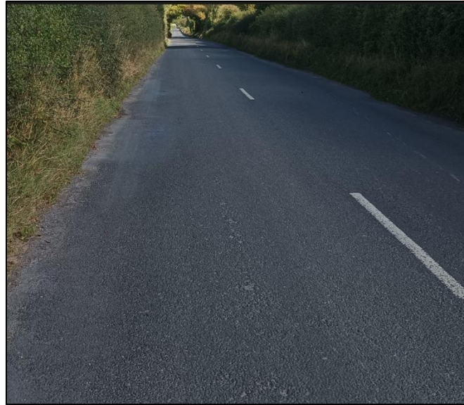
Photograph 26: View North of L1220 Ravelling and Edge Break Up
