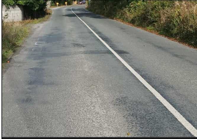
Photograph 3: View North of L1222 Fatting Up on Approach to N69 Junction Area
