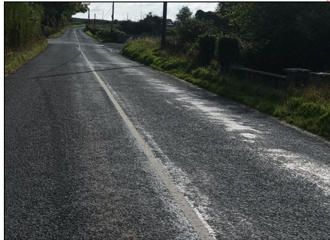
Photograph 6: View South of L1222 Ravelling on Immediate North Side of Greaney Concrete Products
