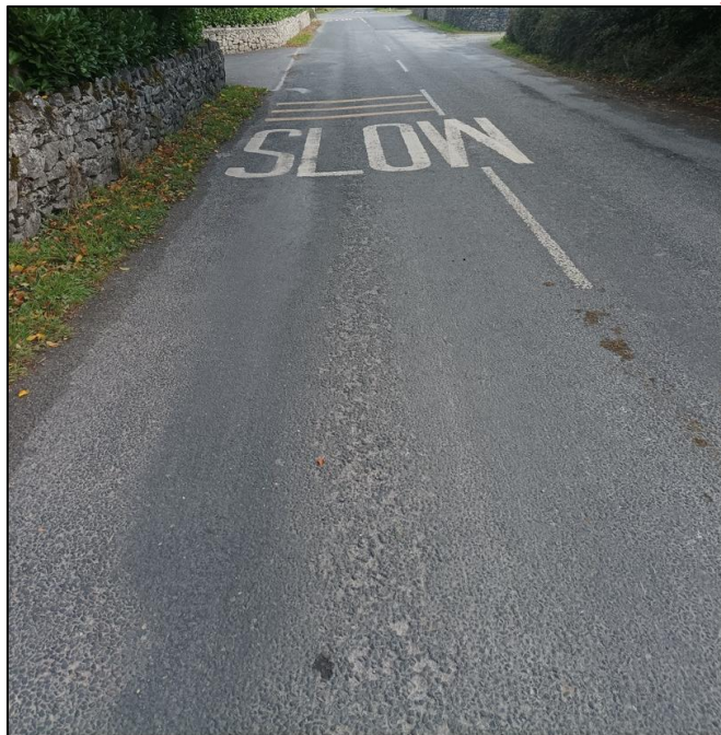
Photograph 22: View North Within Creeves Cross 50 km/hour Zone of L1220 Ravelling
