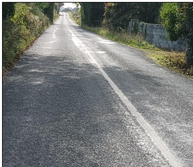
Photograph 2: View South of L1222 Ravelling
